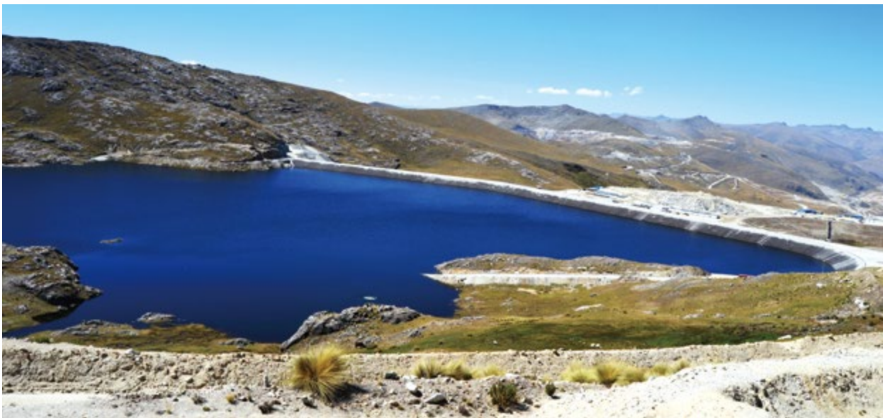
Chuspiri dam at Las Bambas in Peru
